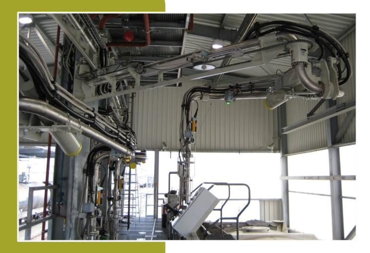
After loading procedure the loading arms can be fixed in idle position by a safety notch. The easy use of **IGATEC Loading Systems** is guaranteed by integrated weight balancing systems. The operating stuff is able to move and position the system with very small effort.
